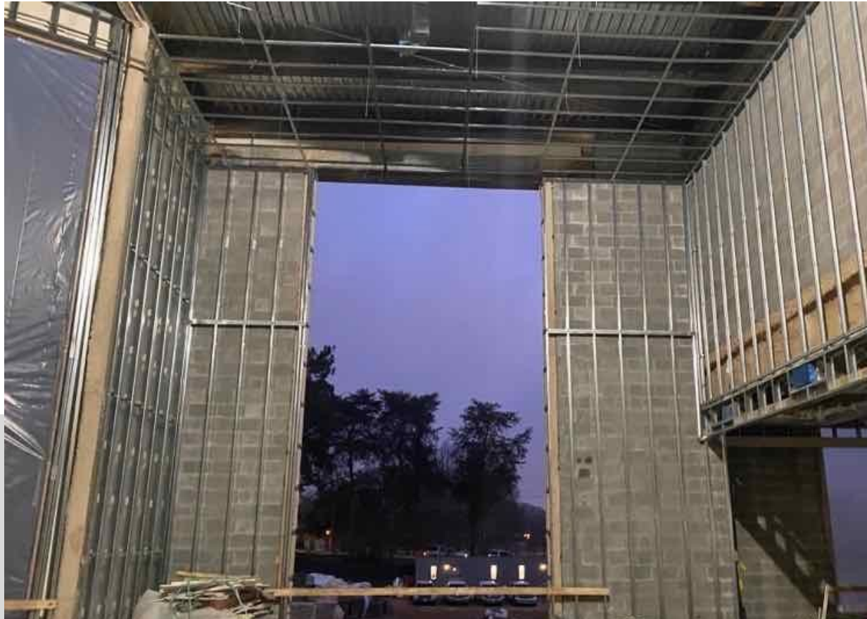
Metal Framing Progress in New Addition Media Center
